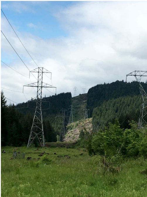
Figure 44 Conditions of Powerline Corridor
